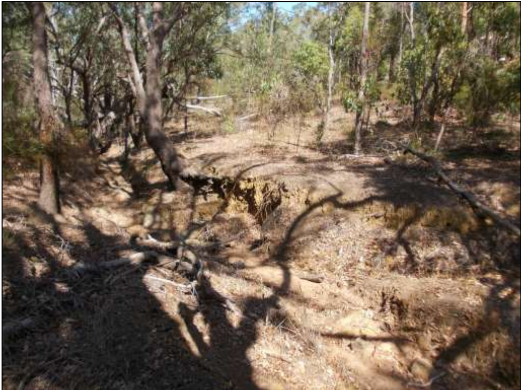
Erosion along creek bed in Mandoon Park
